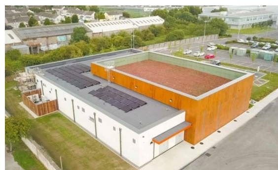
Aerial view of building with green roof on repository and solar panels on office accommodation
