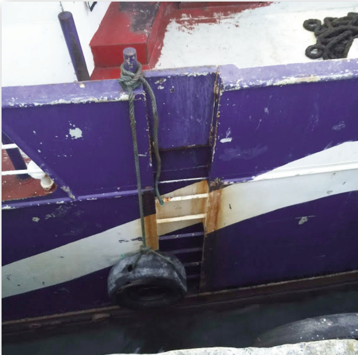
Photograph No. 3. Fixed boarding ladders built in on both sides of the hull of the 'MFV Ellie Adhamh'.
