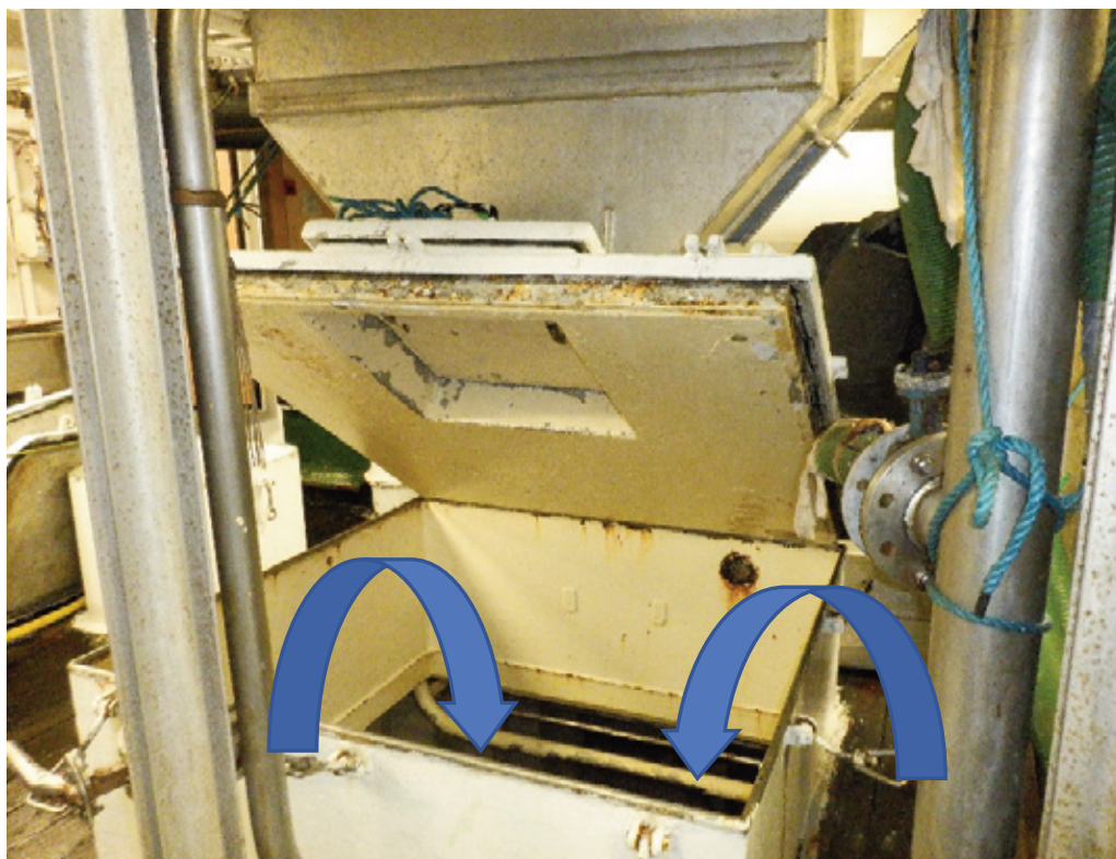
Picture No.9 Main Hatch Opened to Increase Air Flow
