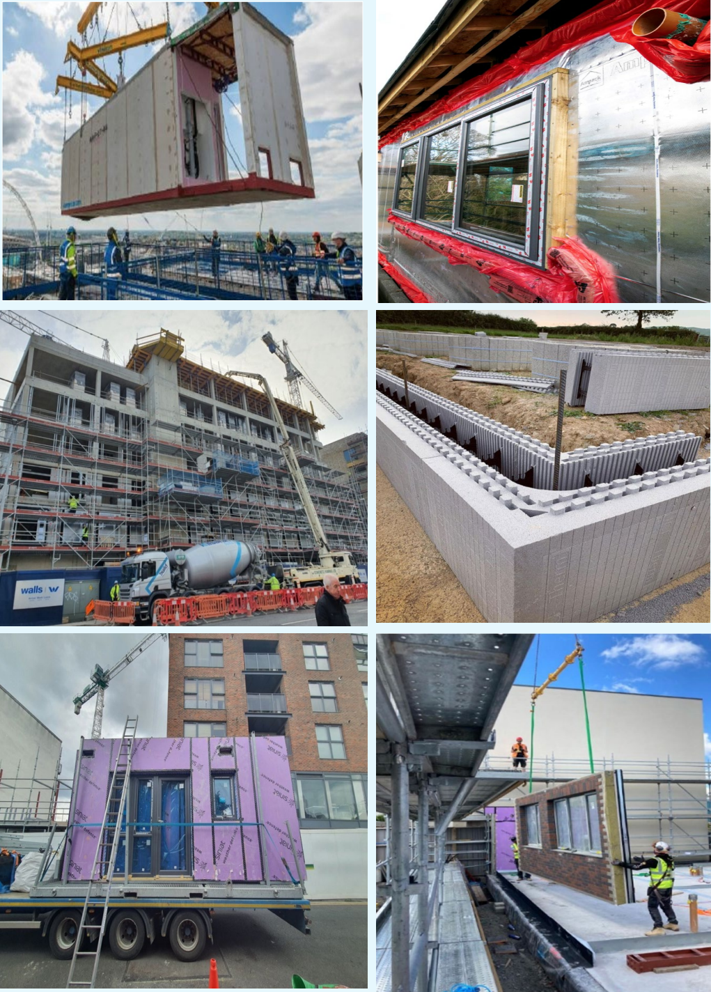
Figure 2.2: Building Examples of Offsite and Near-Site Manufacturing
